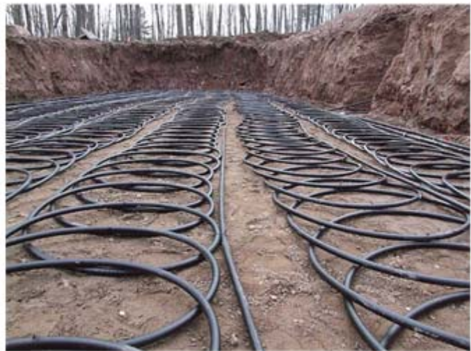
Figure 8: Horizontal Ground Loop
